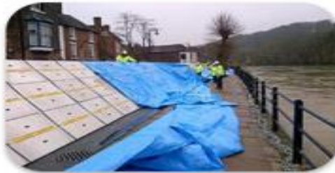
Flood defence / tidal barrage
